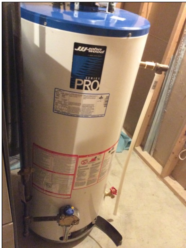
8.6 Item 1(Picture) Hot water tank
