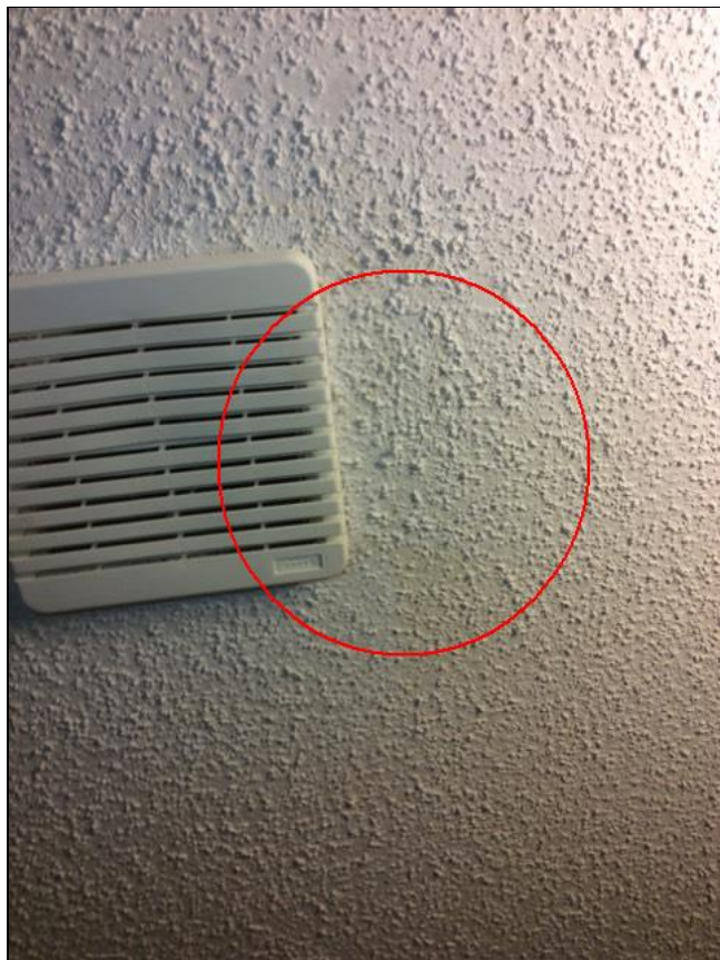
9.0 Item 1(Picture) Moisture stain in second main floor bathroom
