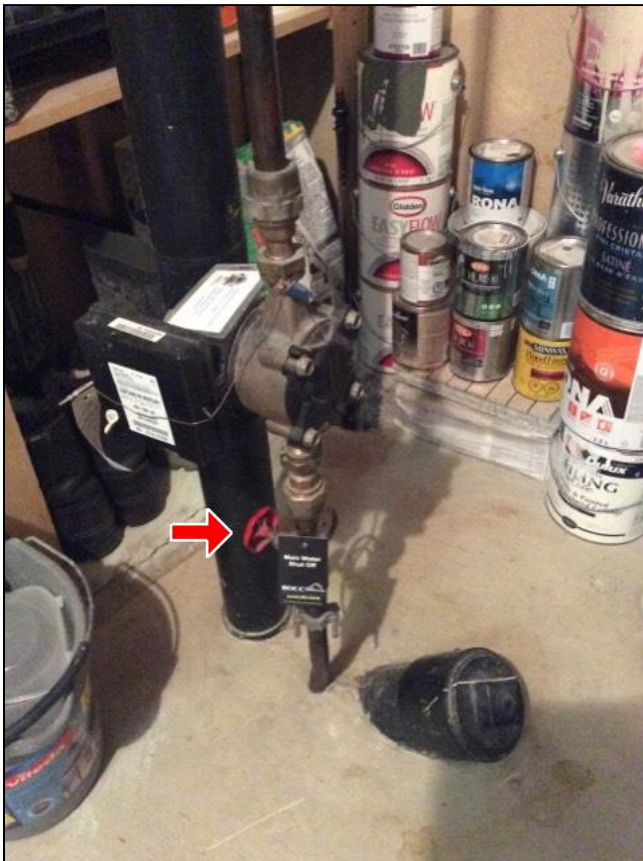
8.3 Item 1(Picture) Main water shut off
