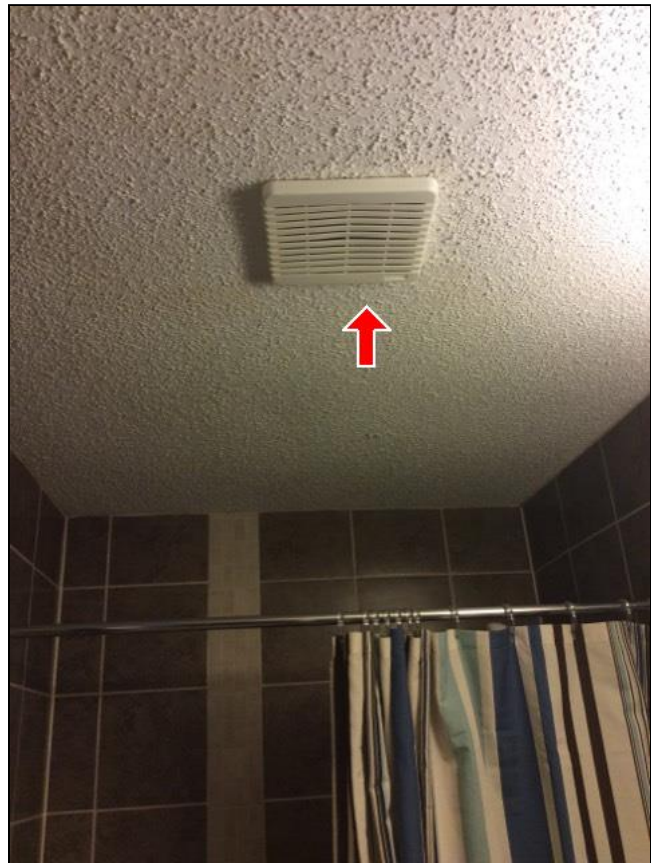
9.8 Item 1(Picture) Second main floor bathroom fan
