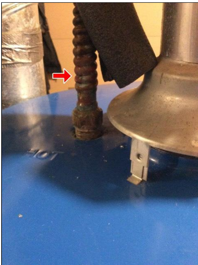
8.6 Item 5(Picture) Water line leaking
