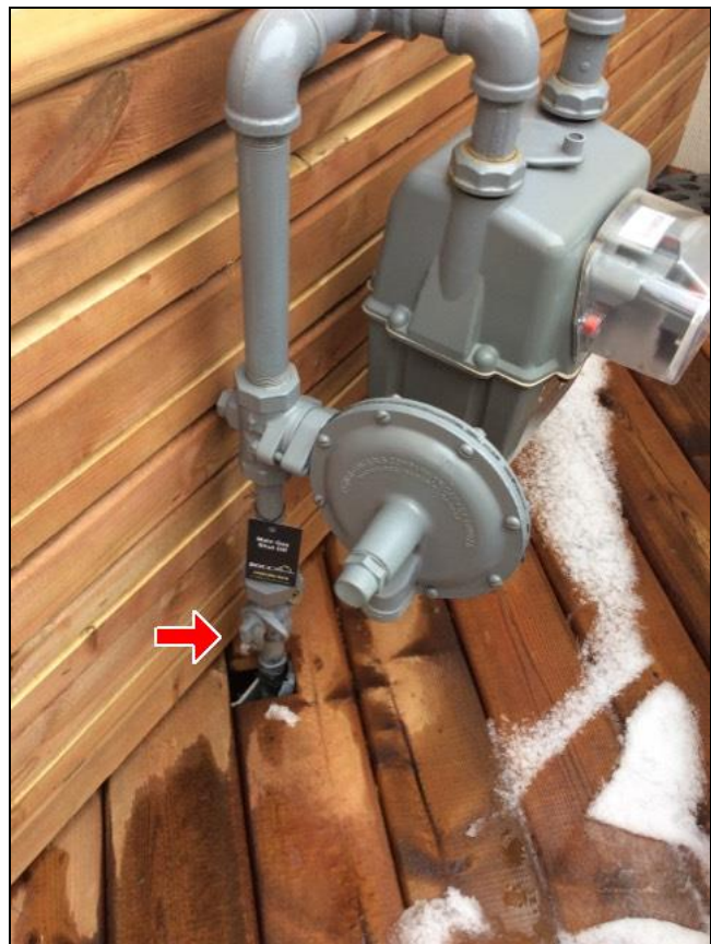
8.5 Item 1(Picture) Main gas shut off
